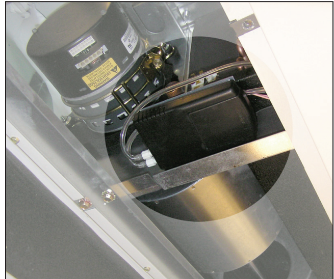
Figure 96: CO 2 Sensor For Demand Control Ventilation
